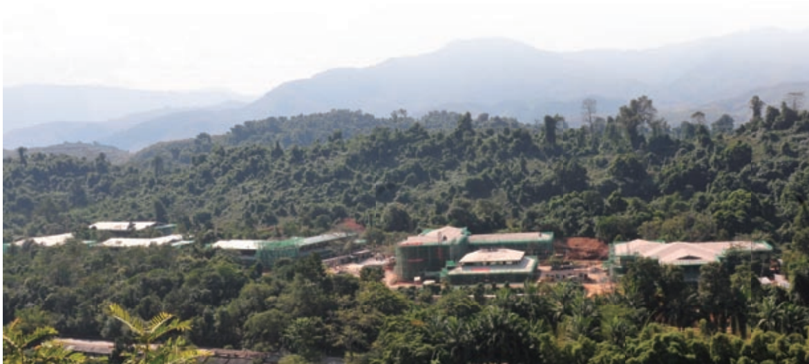
A bird's-eye view of the constructing new research center
